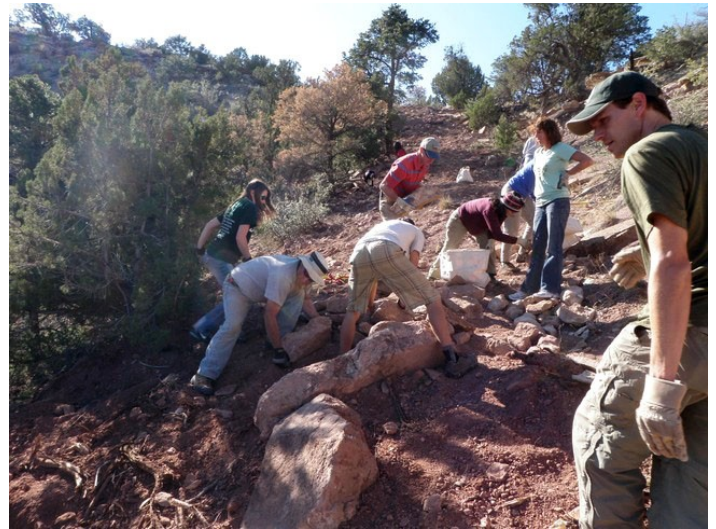
Work Crew Obliterating Road Photo: John Giordanengo
